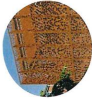
THE LASER-CUT RUSTED STEEL FACADE EXPRESSES THE LOCAL MATERIALITY
