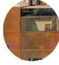
THIS FACILITY WILL BE EXPOSED TO WEATHER AND DISPERSE WITH AGE
